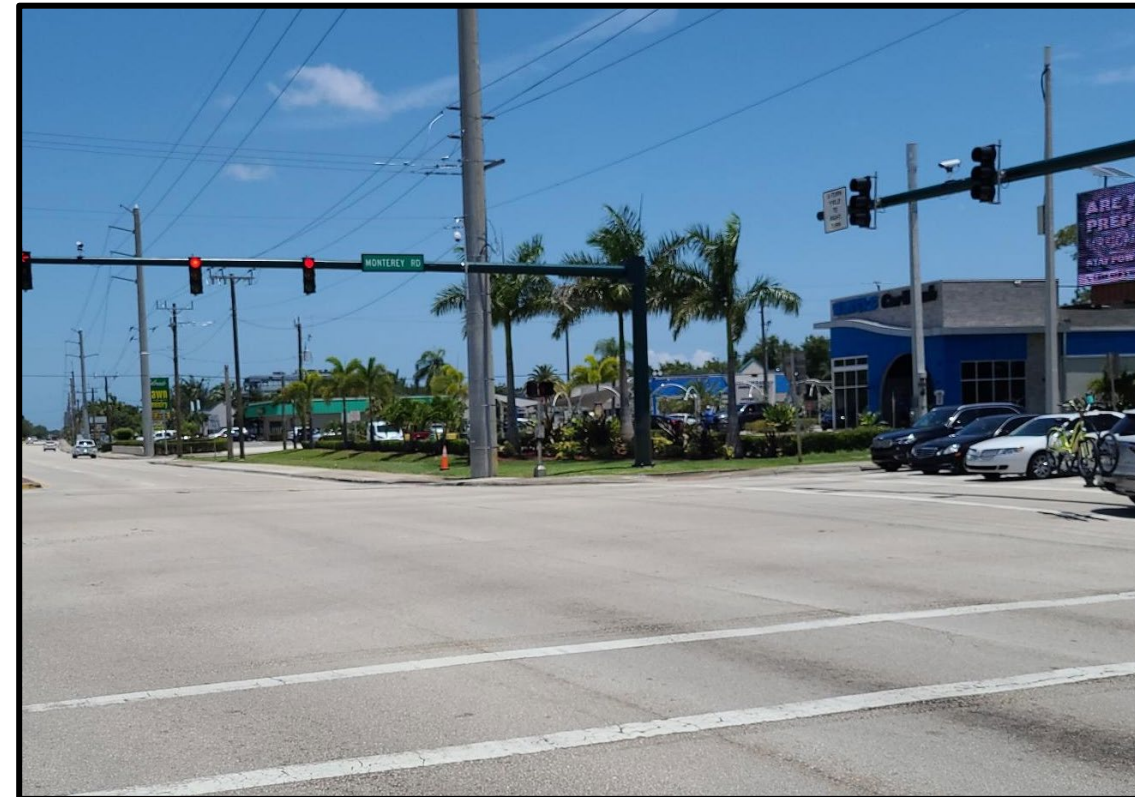
Eastbound SR 76/Kanner Highway at SR 714/Monterey Road (pre-construction)
