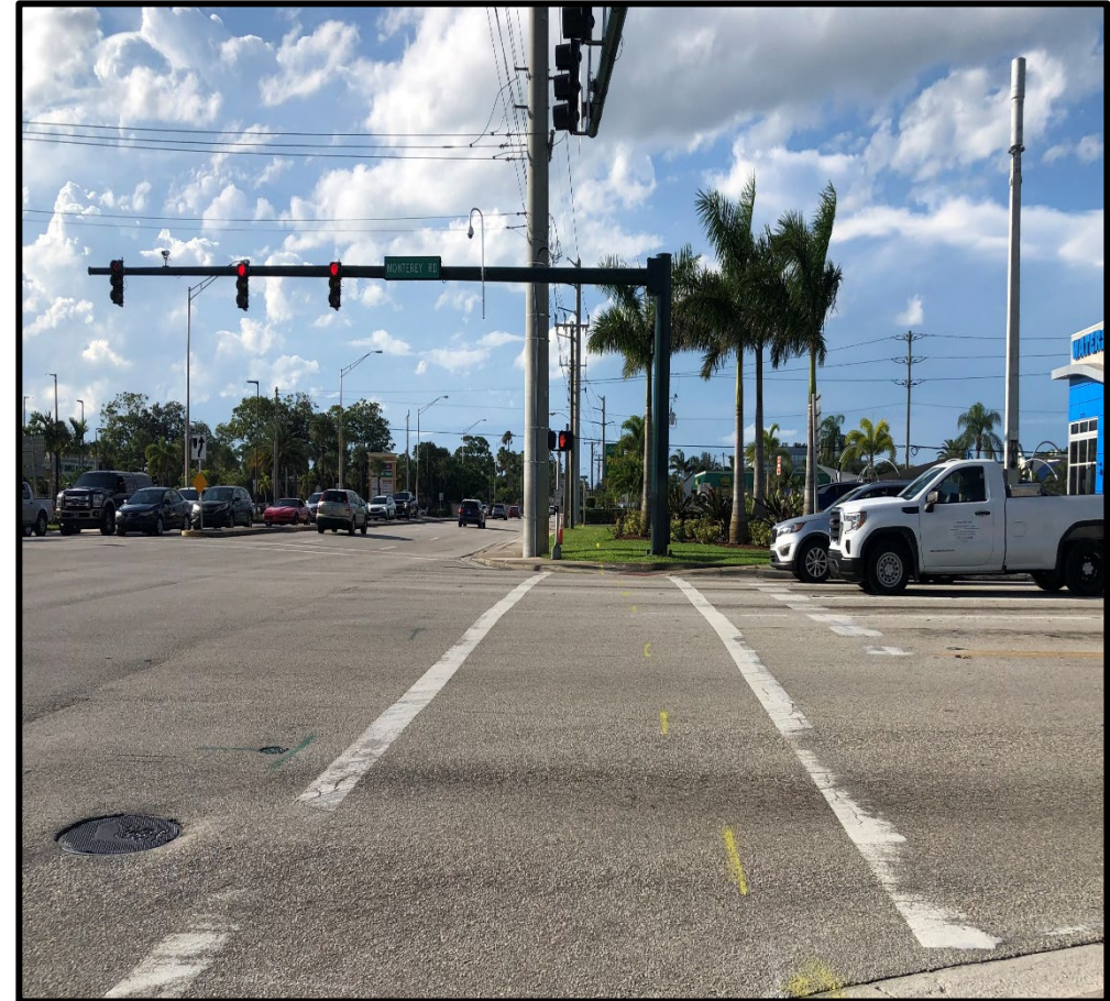
Crosswalk at the intersection of SR 76/Kanner Highway and SR 714/Monterey Road looking north (pre-construction)
