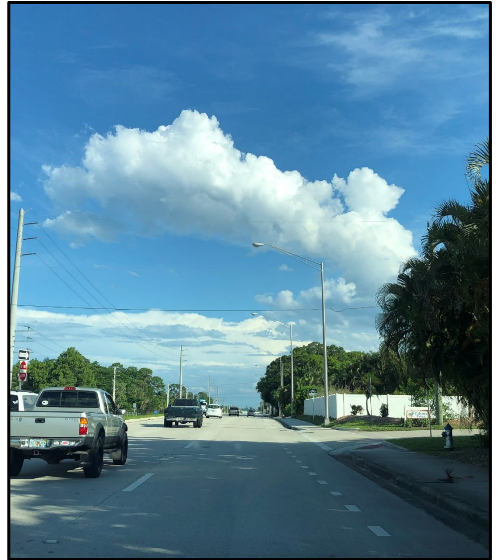
Southbound SR 76/Kanner Highway just north of SW Cabana Point Circle (pre-construction)
