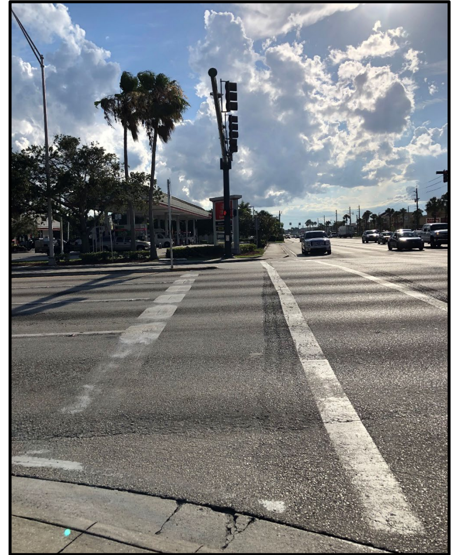
Crosswalk at the intersection of SR 76/Kanner Highway and SR 714/Monterey Road looking south (pre-construction)
