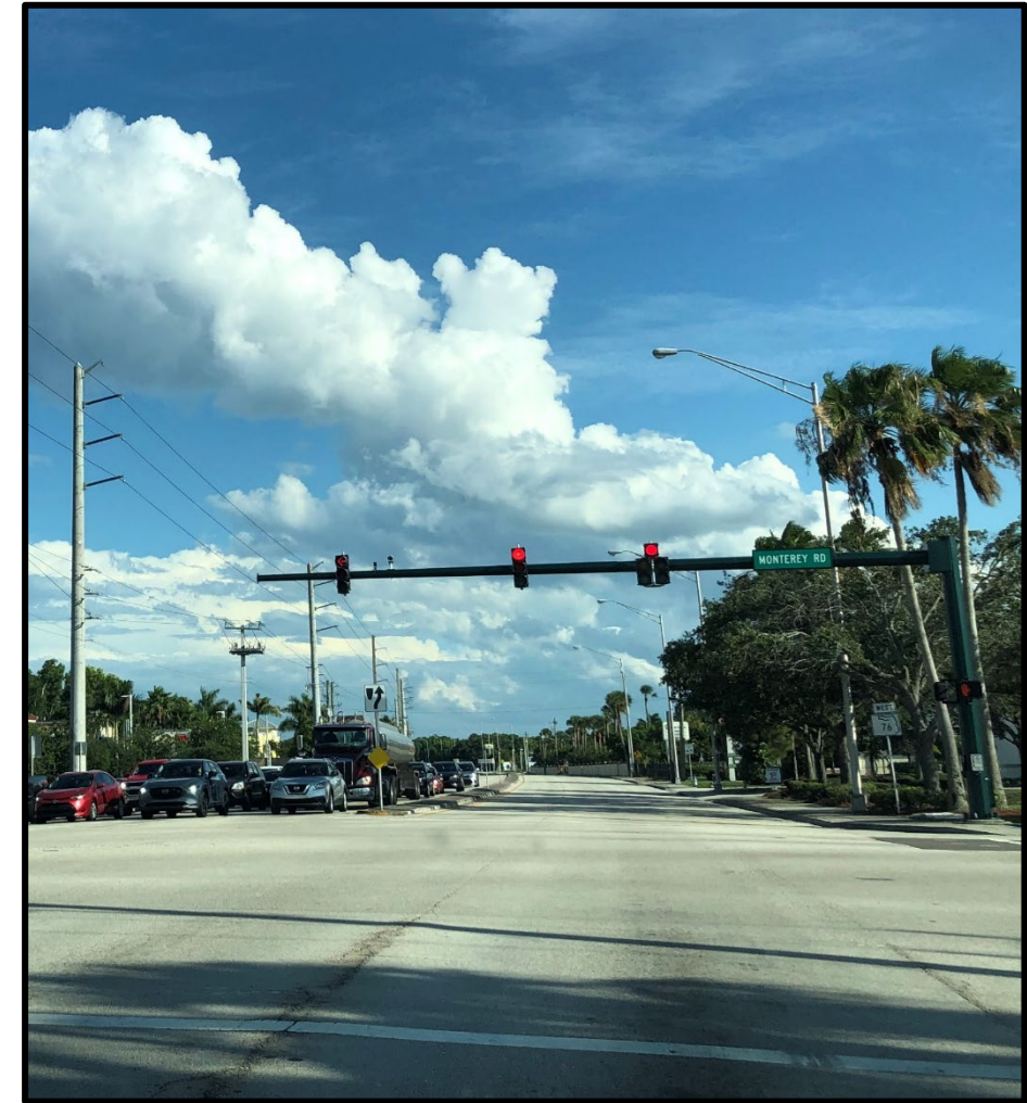
Intersection of SR 76/Kanner Highway and SR 714/Monterey Road heading south (pre-construction)
